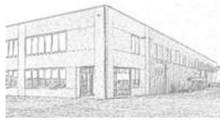
New industrial buildings
