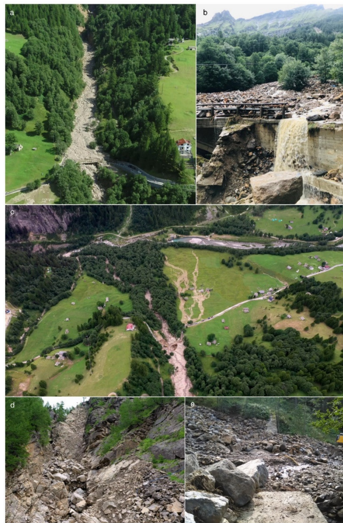
Figure 7. The 12 August 2019 debris flows event along the Croso stream—(a) The bridge covered and filled in below by debris flow accumulation (view taken from the drone video, see along the text); (b) a particular of the left-hydrographic side deviation of the Croso stream active channel (see Figure 6c); (c) view of the earth flows starting down-stream respect to the bridge (view taken from the drone video, see along the text); (d) the up-stream conditions of the Croso stream bed with abundant disrupted deposits (view taken from the drone video, see along the text) (see Figure 6d); (e) a check dam, upstream to the bridge, overwhelmed by debris (see Figure 6c).
