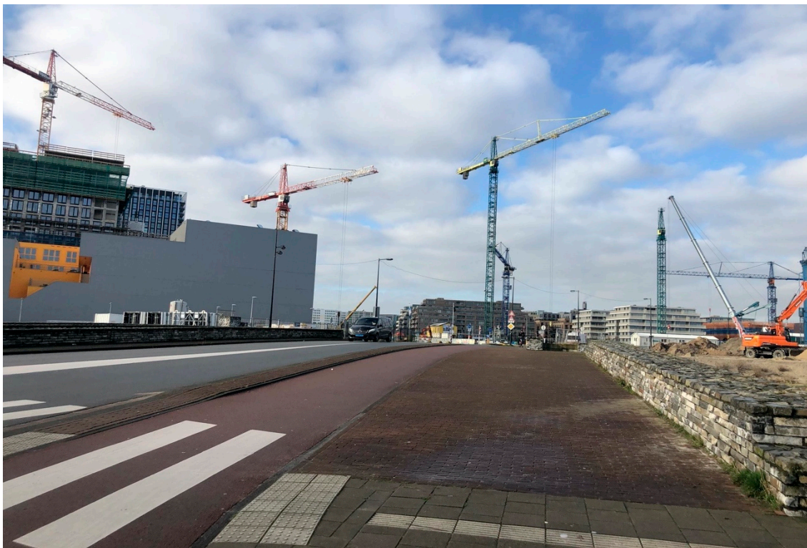
Figure 3. Building work in Buiksloterham.
