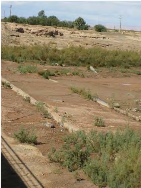
Figure 6. Weirs or dykes are used to slow down the velocity of the river.
