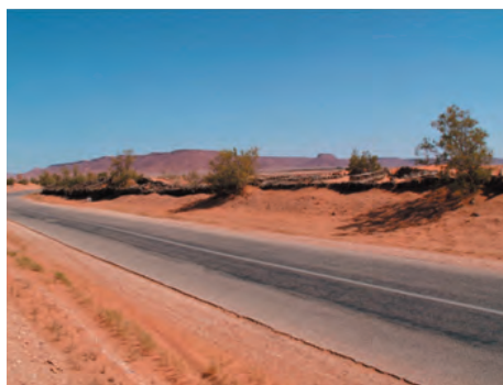
Figure 11. The road Errachidia–Erfoud crossing the « Yerdi corridor », a tract of intensive wind transit, where the road is regularly sandy.
