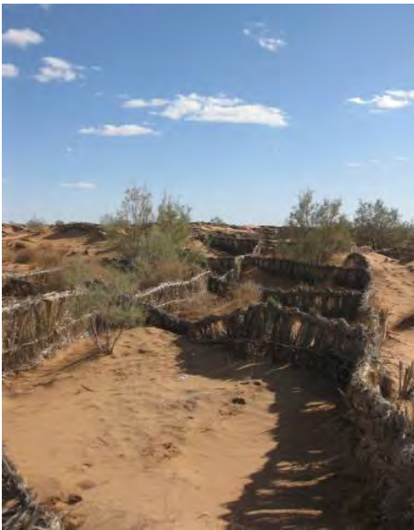
Figure 4. Palm leaf fences are used to prevent sand encroachment.
