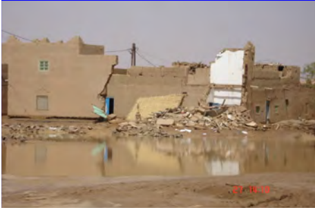
Figure 2. Collapsed houses in Merzouga.
