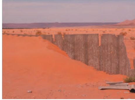
Figure 12. Cement fences erected in 1981 are broken and buried in sand (N31°32'80 O4°10).
