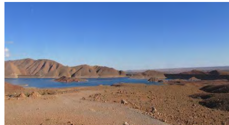
Figure 5. The Hassan Addakhil Dam and its water reservoir 28.10.2011.
