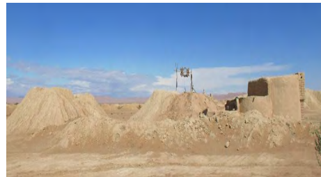
Figure 7. Abandoned khattara with its two sandy wells and an access to the underground canal in Errachidia 27.10.2011.
