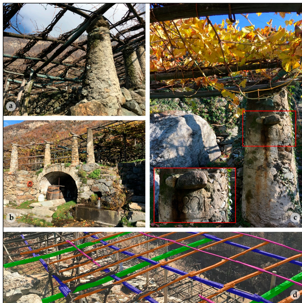
Figure 7. (a) Historical vine-breeding technique: pergola made of chestnut poles supported by stone columns. (b) Pergolas integrated with other important historical landscape elements of rural architecture. (c) Dated stone columns for pergola support (1821). (d) Detail of four orders of chestnut poles perpendicularly overlapped that make up pergolas (shown in green, blue, orange, and pink).
