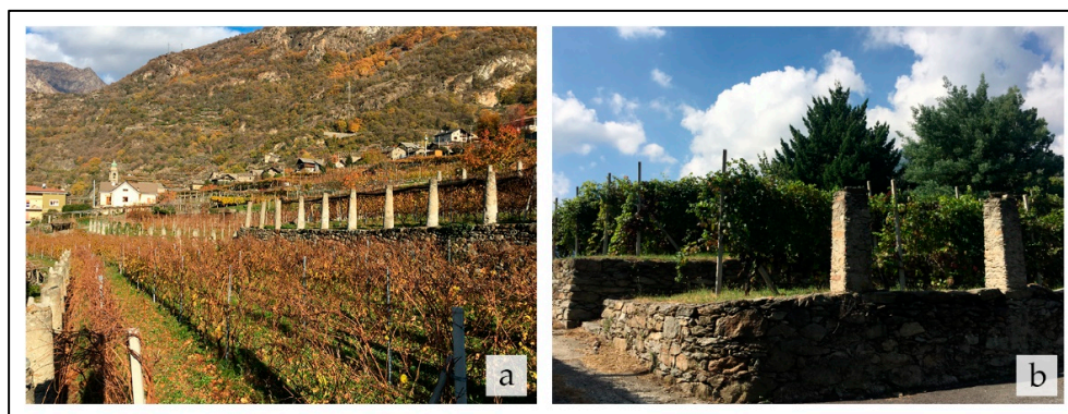
Figure 11. (a) The introduction in the lower part of the slopes of the espalier vine-breeding technique in place of the traditional pergola caremiese, which causes a loss of the landscape's integrity. Additionally, the stone columns once used for the support of pergolas remain but have lost their role. (b) Detail of terraces where the historical vine-breeding technique was changed causing the loss of the landscape's integrity.
