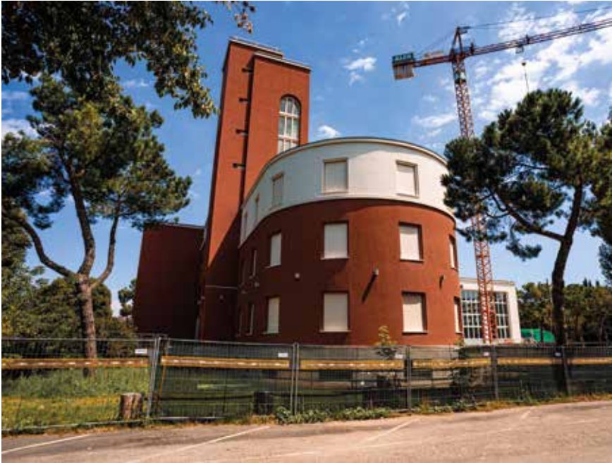
Figure 3. The headquarters of Opera Nazionale Balilla (ONB) under restoration in August 2014. Picture by G. Casa.
