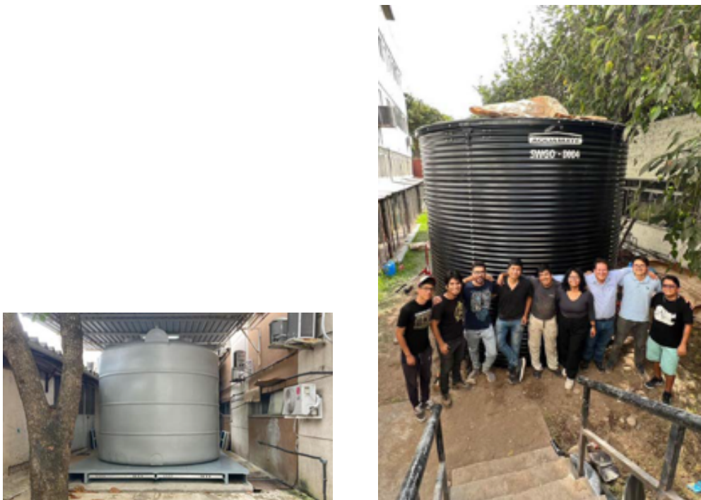
Figure 1. Tanks prototypes: roto-moulded tank installed at CBPF Rio De Janeiro (left panel) and steel tank mounted at Arequipa University (right panel).
