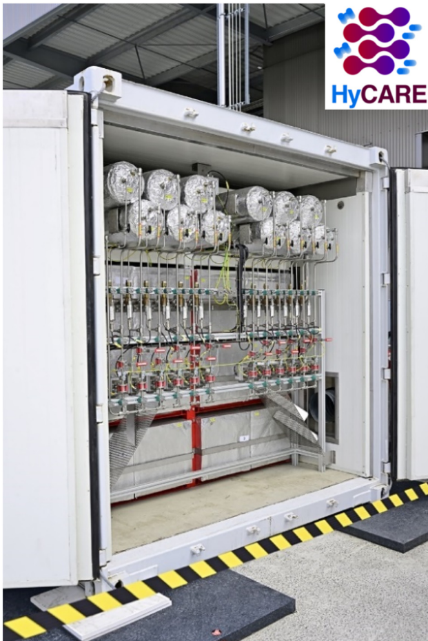
Fig. 4: Hydrogen storage system developed in HyCARE project: Cylinders at the top contain the metal hydride for hydrogen storage and boxes at the bottom contain the PCM for heat storage.
